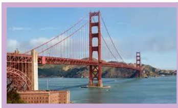
7. Golden Gate Bridge, US
